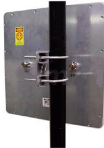
Figure 31. Installing Flat Panel Antenna to the Pole
